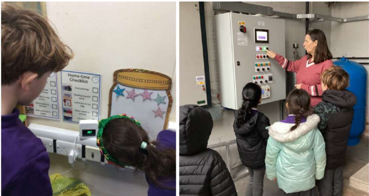
Above: After investigating classroom temperatures, Horsford's Eco Team worked with their headteacher to adjust heating timings.
